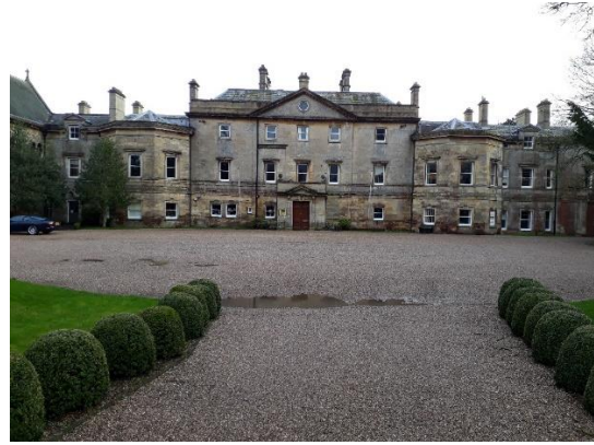
View of Wellingore Hall Entrance Front
